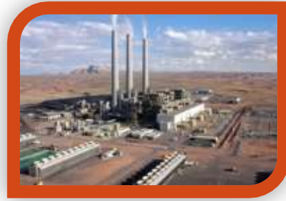
Navajo Generating Station, Page, AZ
